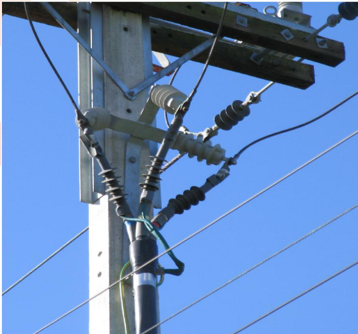
Cable Termination with Lightning Arrestors
