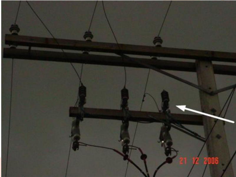
Cable Termination with Lightning Arrestors
